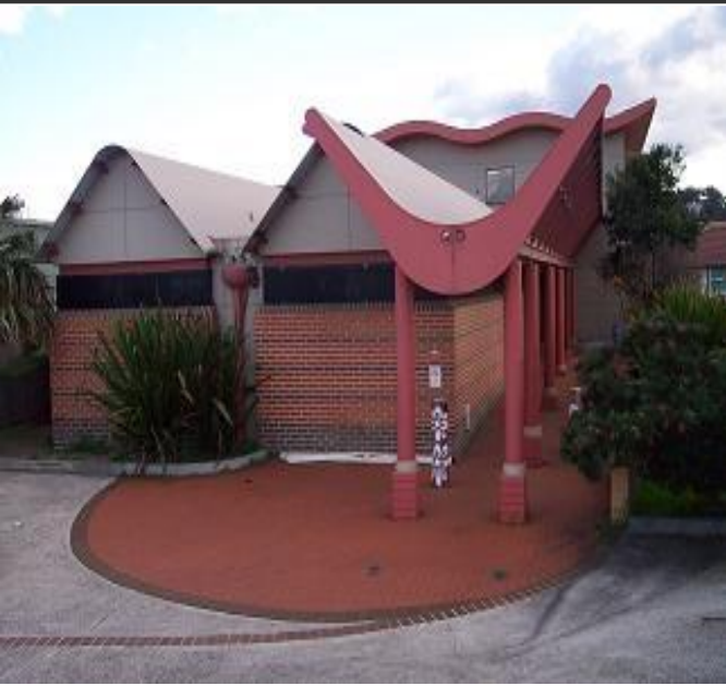
Wollongong 150 Church Street
