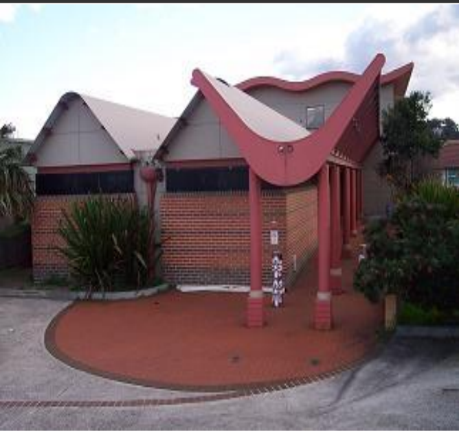
Wollongong 150 Church Street
